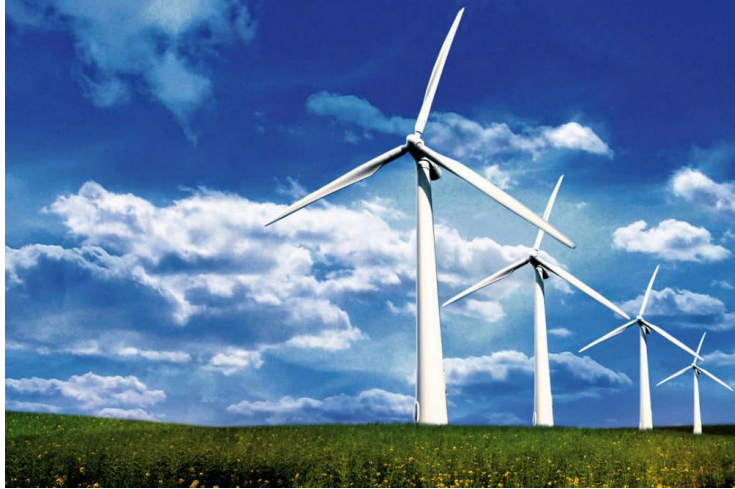
Rotor speed detection of a wind turbine
